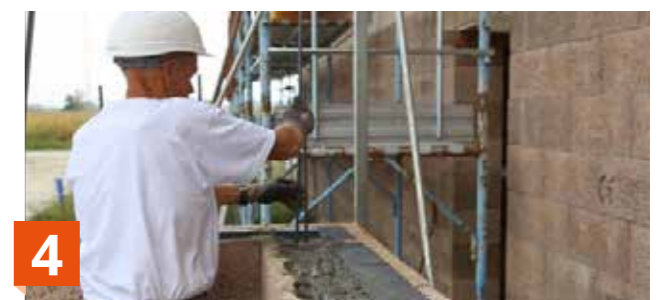
4 Fresh casting insertion of vertical seismic steel reinforcements
