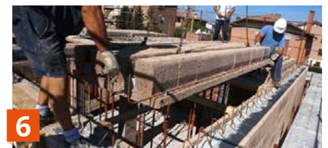
6 Laying of the floor slabs, calculated and made to measure.
