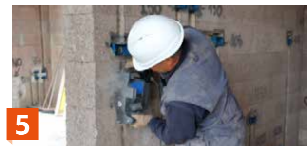
5 Chasing of wall with a router
