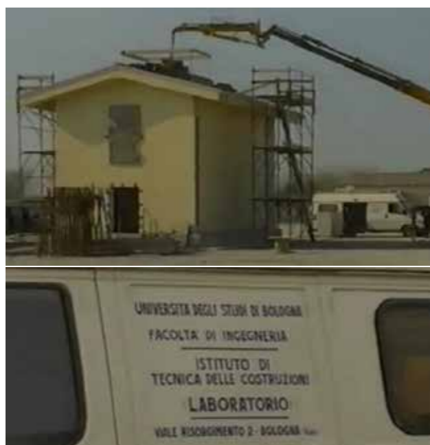
Building constructed with Isotex blocks and panels, tested with the Vibrodina of the University of Bologna.
