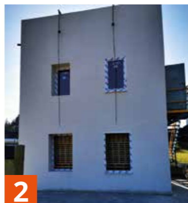
2 The Isotex wall had 2 openings on the ground floor and 2 on the first floor, plus a rib without openings at the top
