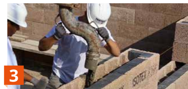
3 Filling of the blocks with concrete (every 6 rows)
