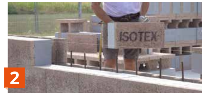
2 All subsequent rows laid dry
