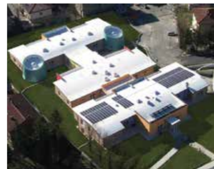
Pavullo school complex (MO) - Italy
