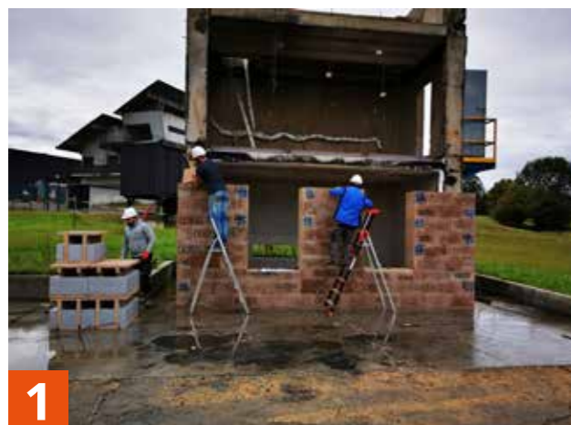
1 A 5.5x7 metre wall was built with a 44/23 Basf-Neopor® graphite block
